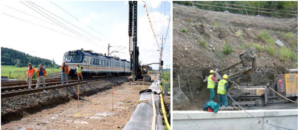
Fig.6 The Installation of lime-cement columns (left) and soil nailing (right) for substrate stabilisation (INNTRACK project [3])
