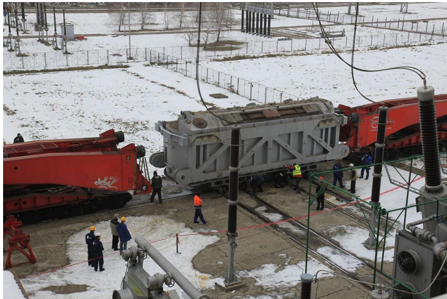
Fig.3 Transformer 725 MVA on the loading position for the “Schnabel” wagon at thermal power plant TENT B in Obrenovac
