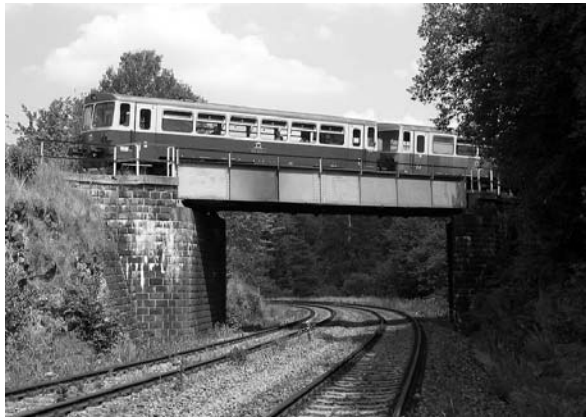
Fig. 5 Risk place on transport infrastructure
