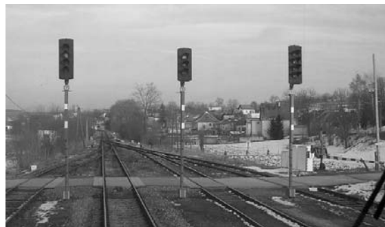
Fig. 3 Station interlocking plant
